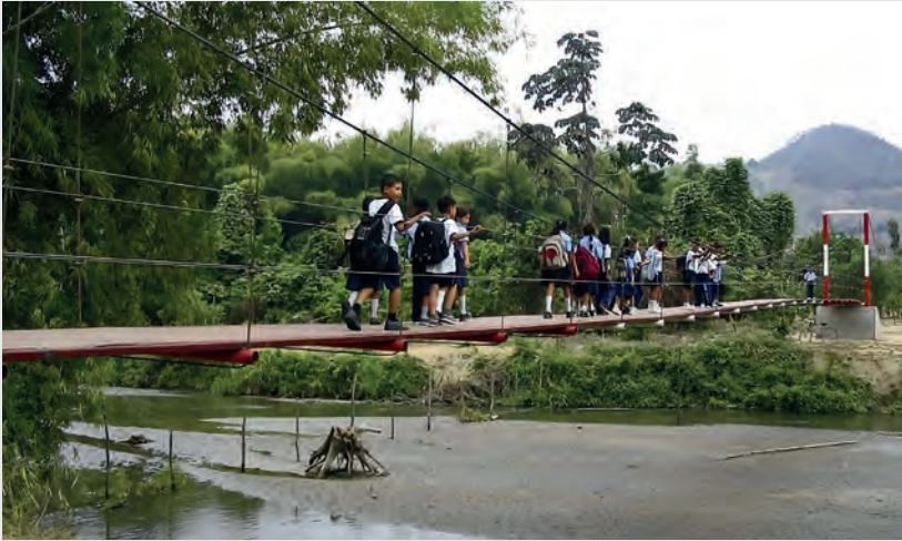
More than 2.5 million people have benefited from the bridges.
